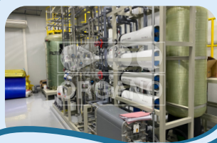
Project name: Water for injection Location: Quang Minh IP, Hanoi Year of completion: 2020
