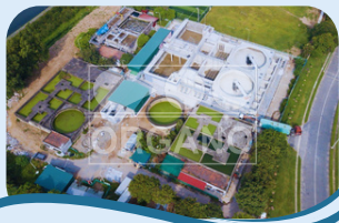
Project name: Sewage treatment plant Location: TLIP I, Dong Anh Capacity: 11,000m3/day Year of completion: 2019
