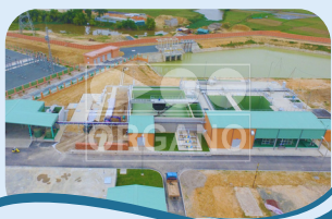
Project name: Sewage treatment plant Location: TLIP III, Vinh Phuc Capacity: 3,000m3/day Year of completion: 2019
